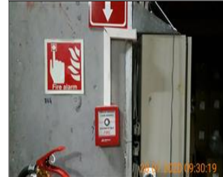
Photo of fire safety equipment FIRE ALARM BUTTON.jpeg
