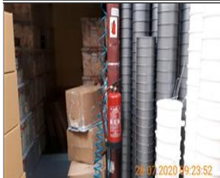
Photo of fire safety equipment FIRE EXTINGUISHER.jpeg
