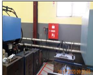
Photo of fire safety equipment FIRE HOSE CABINET.jpeg
