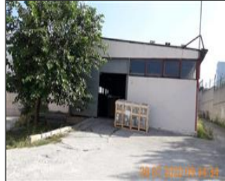
External photo(s) of the production unit(s) WAREHOUSE BUILDING.jpeg
