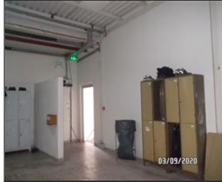
Photo of the inside of the main production hall Dressing room.JPG
