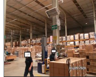
Photo of non-conformity NC7.25and7.1-PARTIALLY CORRECTED-Portable heaters were fixed to upper panels in working stations.JPG
