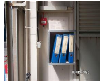
Photo of fire safety equipment NC7.14-CORRECTED-Fire alarm button in the chemicals storeroom.JPG
